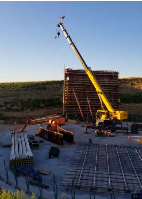
City of Tracy 3.75 MG Water Tank Tracy, CA
