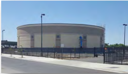
3.0 MG Water Tank Tracy Hills, CA
