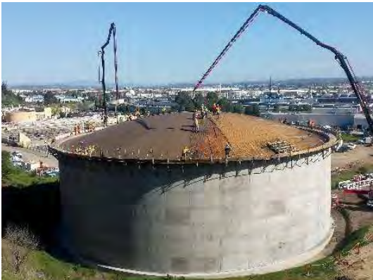
Freespanning Concrete Dome Construction
