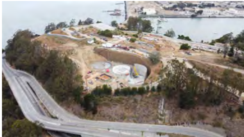
San Francisco Public Utilities Commission 3-1.34 MG Water Tank San Francisco, CA
