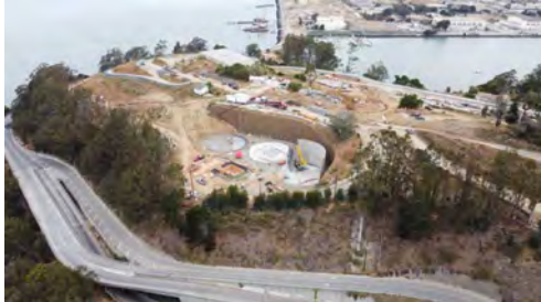
San Francisco Public Utilities Commission 3-1.34 MG Water Tank San Francisco, CA
