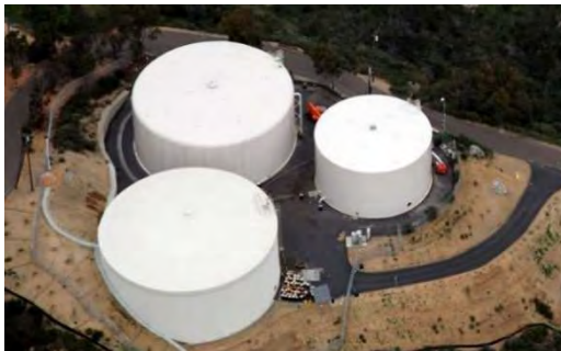
Location: Jamul, CA Year Completed: 2009 Project: 2.0 MG Ground Storage Tank Owner: Otay Water District DN Tanks Scope: General Contractor Engineer: By Owner – Otay Water District
