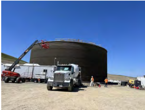
Lennar Homes of California 2.67 MG Water Tank Tracy Hills, CA
