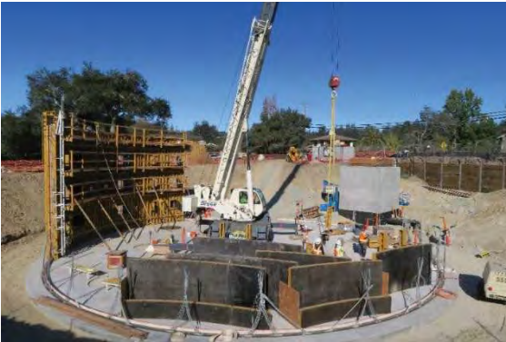
Floor Slab and Corewalls
