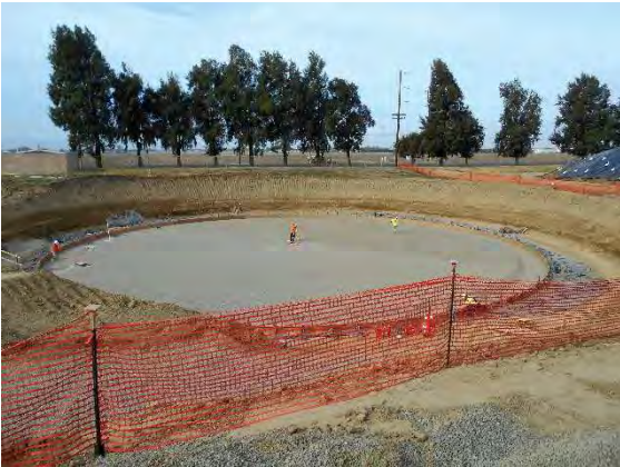
Tank Site Preparation
