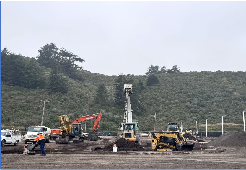
Excavation and ground improvement in Progress for Building Foundation
