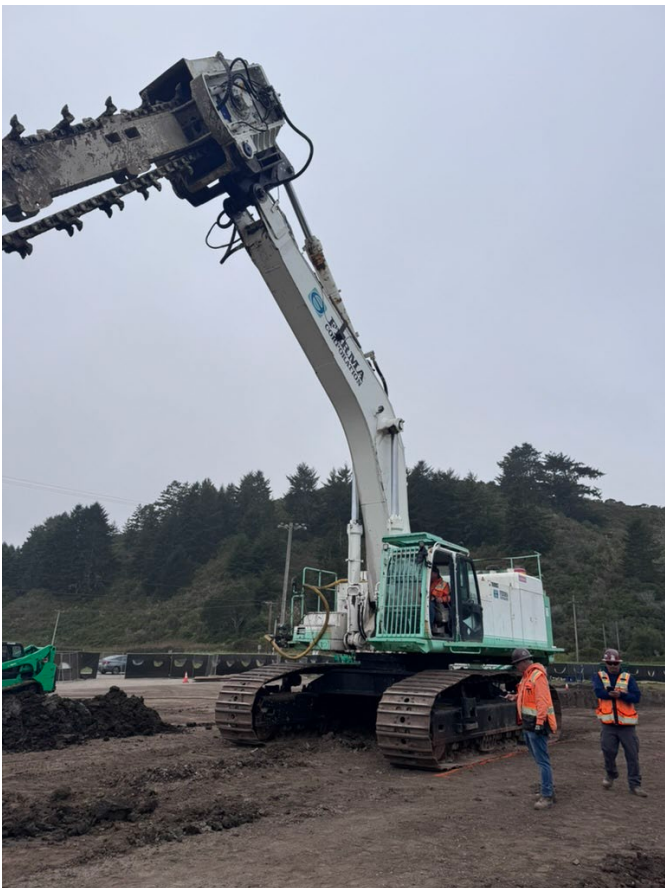
Excavation and ground improvement in Progress for Building Foundation
