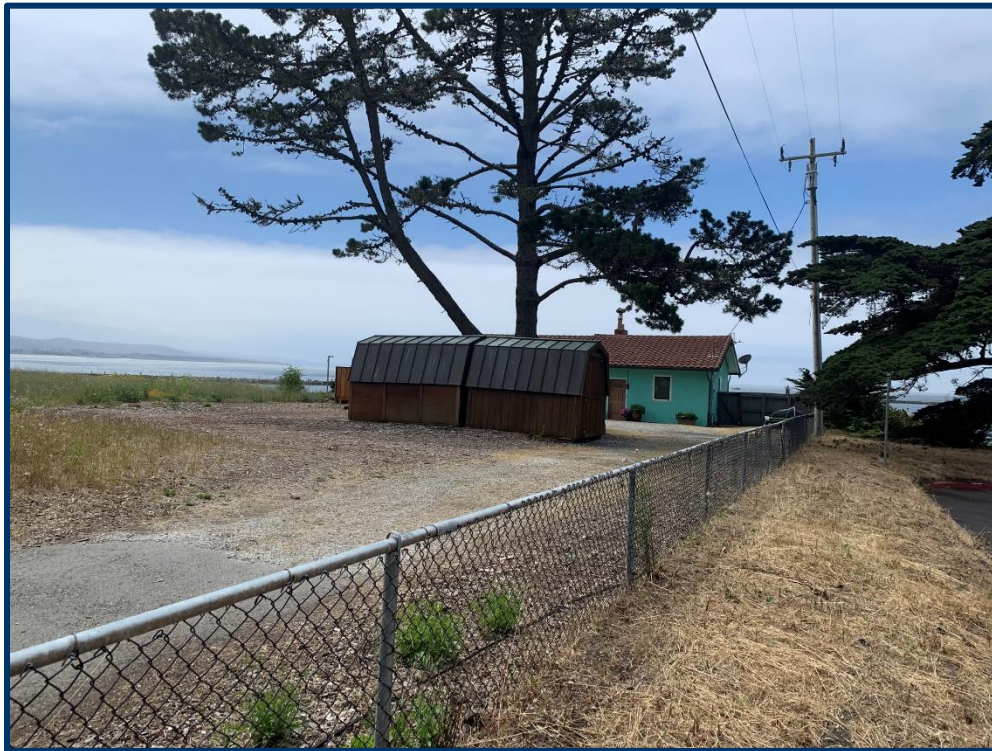
View of APN -390 with view of the house improvements
