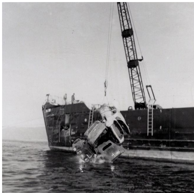
Figure 9. Car bodies being placed on Ventura Artificial Reef in 1960.
