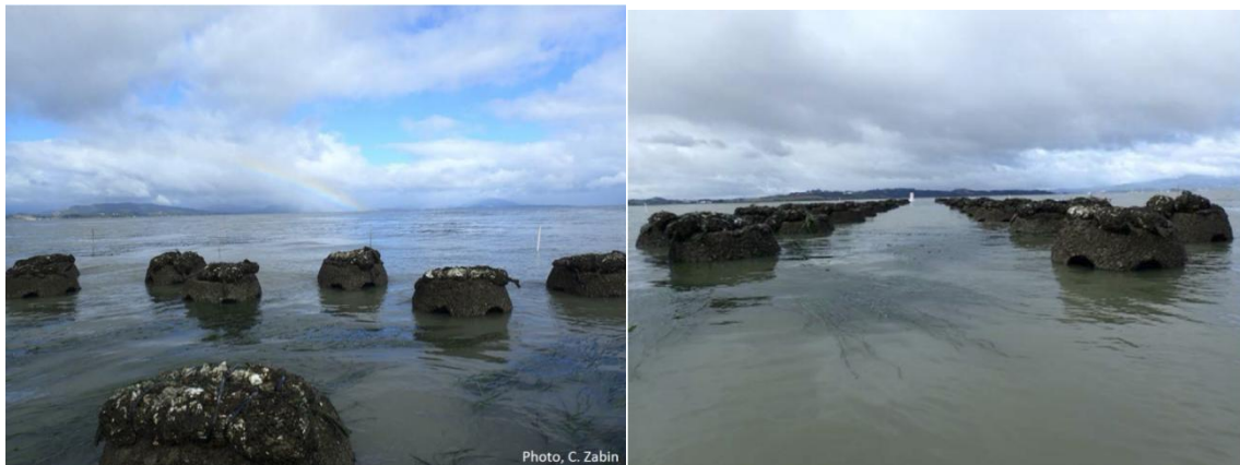
Figure 11. Reef Ball elements constructed of baycrete with oyster shell bags on top, Giant Marsh. Source: Boyer et al. (2020). 143
