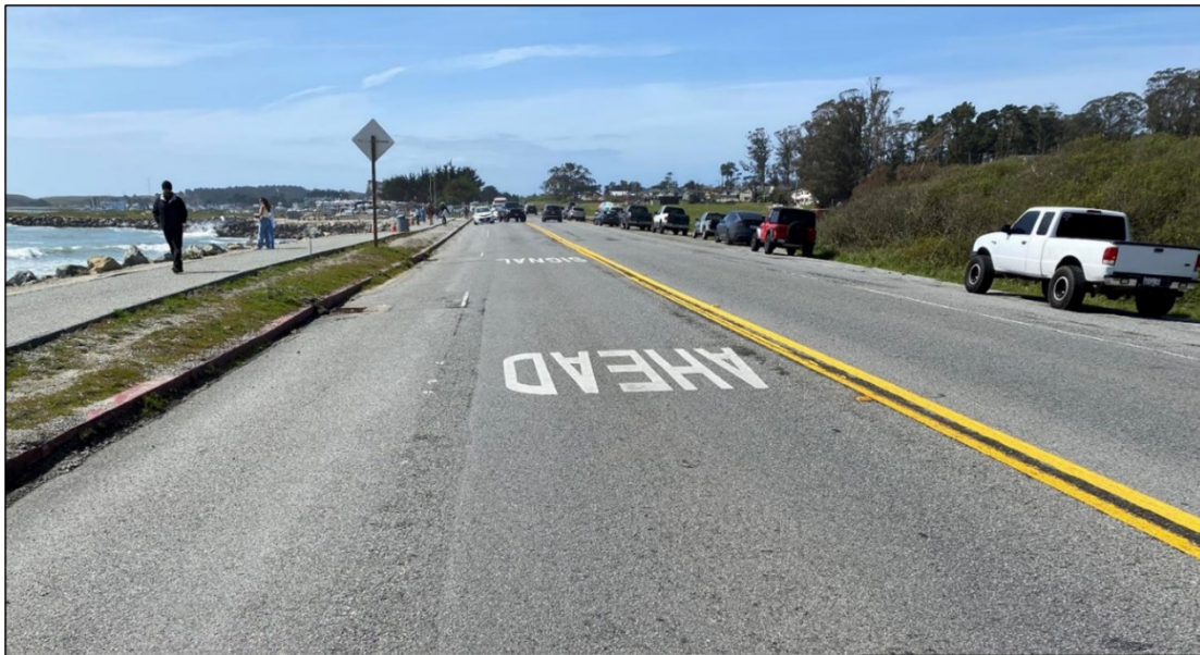
Figure 4 Existing Conditions on SR 1
