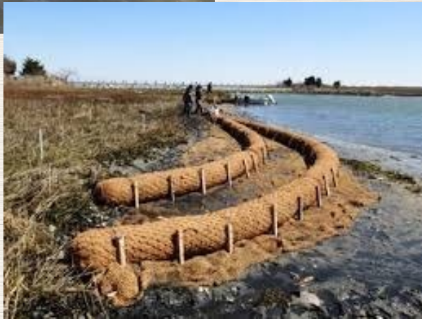
Coir Fiber 'Nature Based' Revetment
