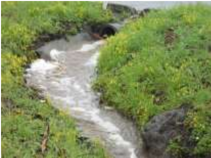
Photo 13 - Larger Park stormwater flow flooding from pseudo storm drain under the eastern side of The Alameda to open-air ditch in its median
