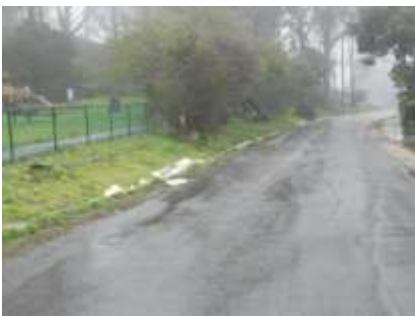
Photo 04 - Diverted lesser Park stormwater flow flooding down Columbus (towards Santiago)
