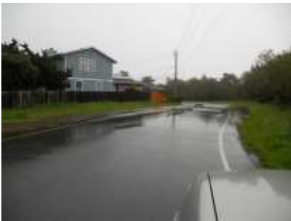
Photo 66 - Pooling runoff flooding the entire roadway at the curved portion of Sonora (towards the storm drain)
