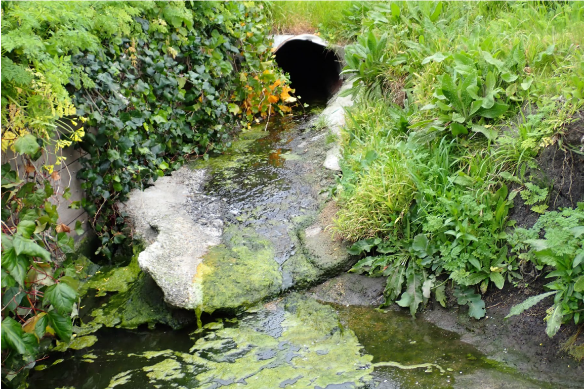
Figure 27 Poured concrete apron at 2805 Naples Ave
