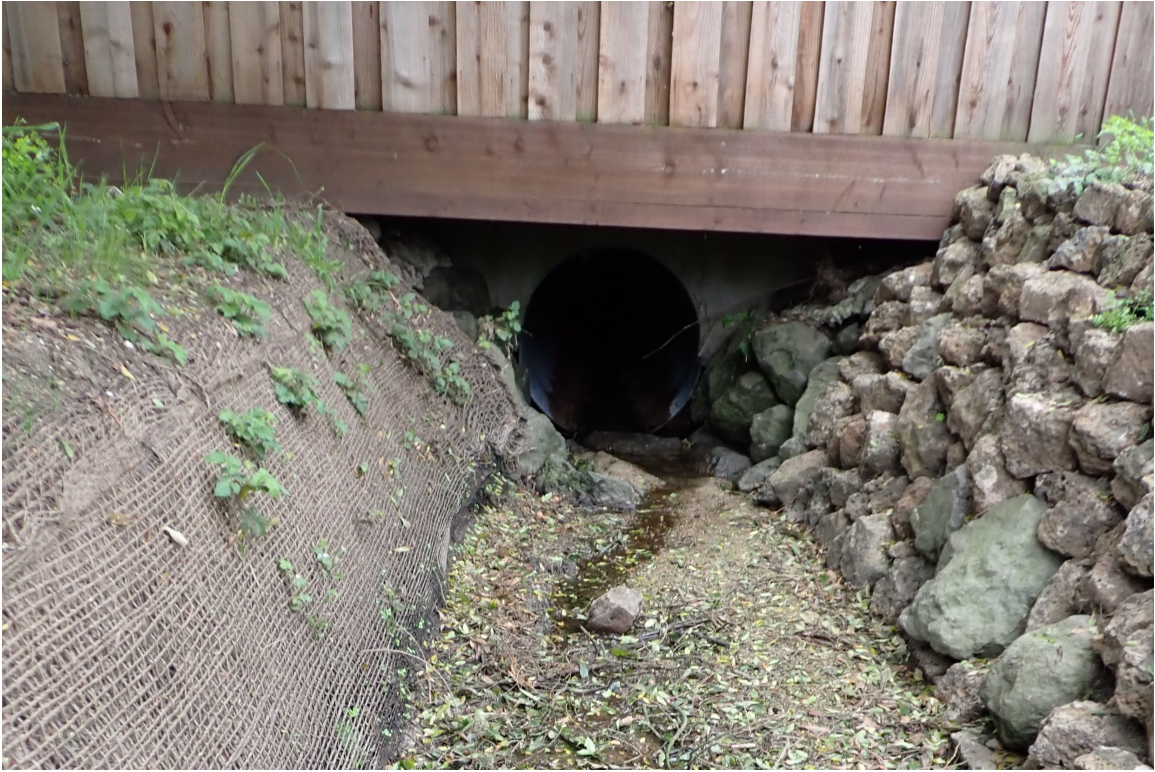
Figure 7 Inlet to 36" culvert under 2805 Alameda Ave
