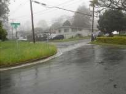
Photo 37 - Additional flooding continuing down from Ave. Portola over the intersection with The Alameda
