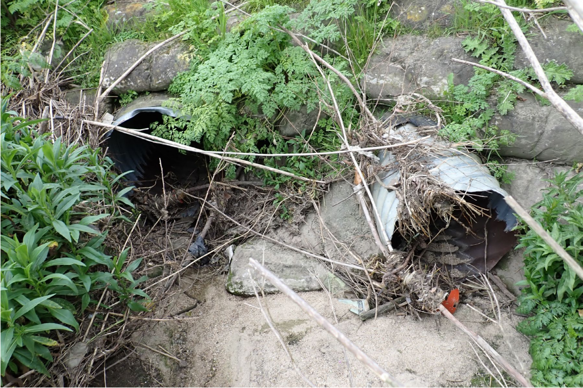
Figure 16 Inlet to parallel 17" and 24" culverts under Coastal Trail
