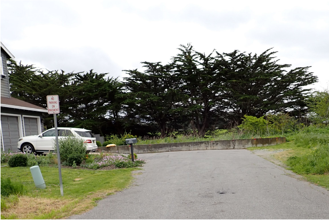
Figure 25 Concrete barrier at end of Alameda Ave
