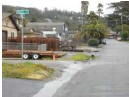
Photo 61 - Flooding down Sonora over x-street Madrid (towards Ave. Granada)
