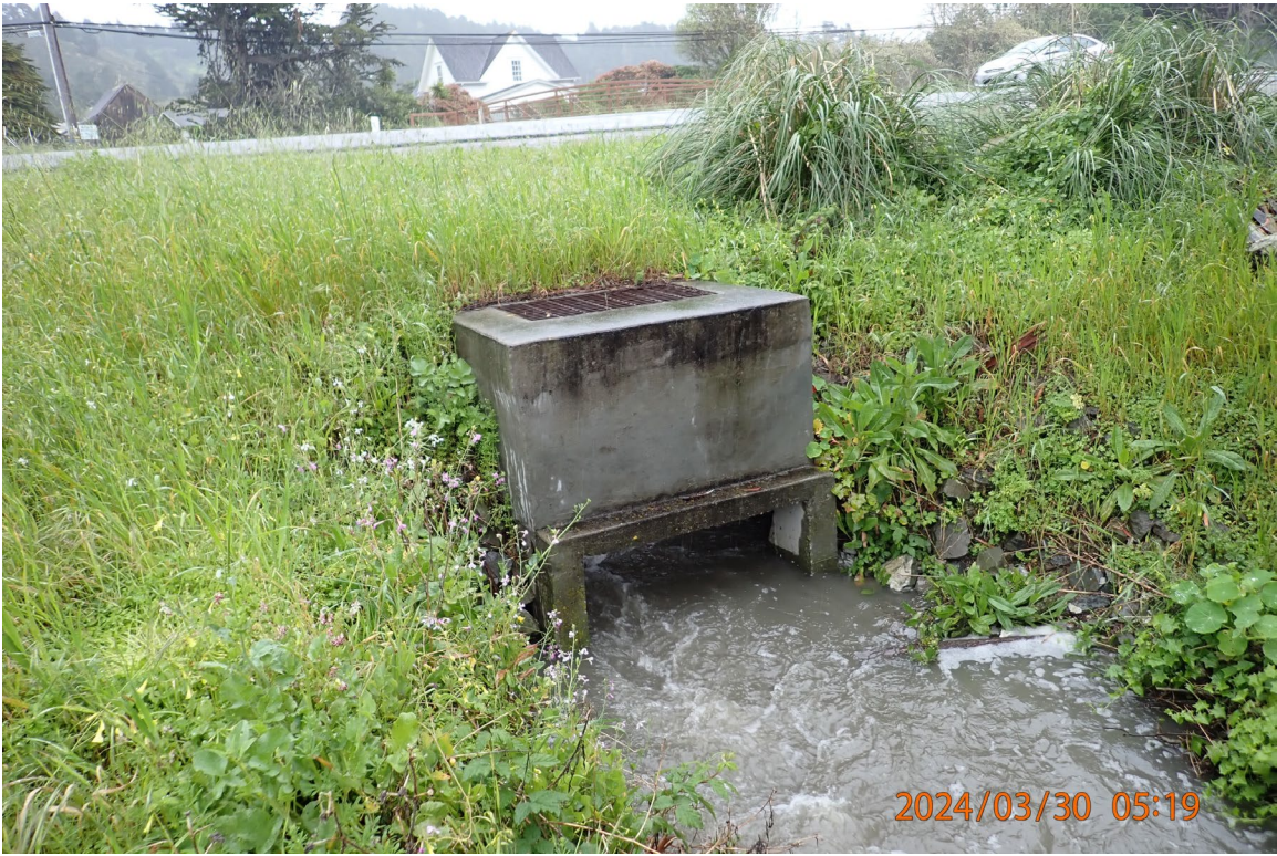
Figure 5 Outlet from the two parallel 25" culverts under Highway 1
