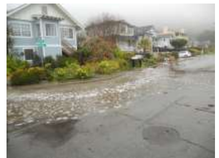
Photo 06 - Diverted lesser Park stormwater flow flooding into pseudo storm drain at intersection of Columbus & Santiago then under street to meadow below
