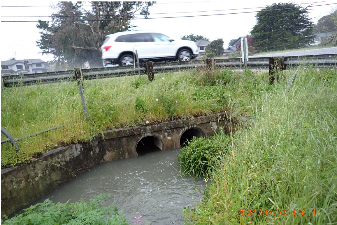
Figure 3 Inlet to parallel 25" culverts under Highway 1
