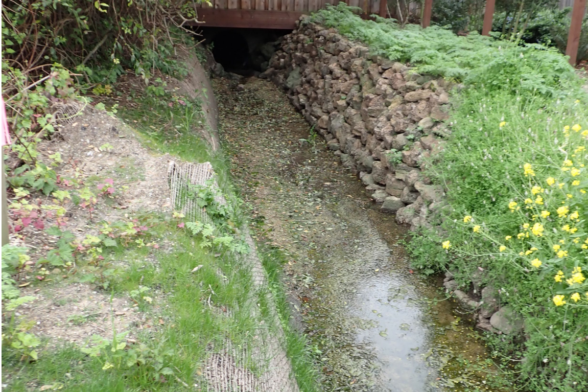
Figure 30 Trapezoidal channel with riprap and jute netting at Rossi Residence
