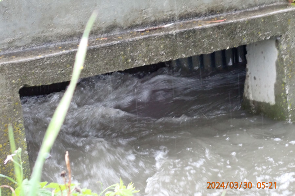
Figure 6 Outlet from the two parallel 25" culverts under Highway 1
