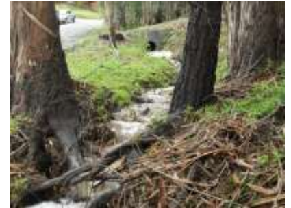
Photo 28 - Deep open-air ditch down Ave. Portola from Columbus
