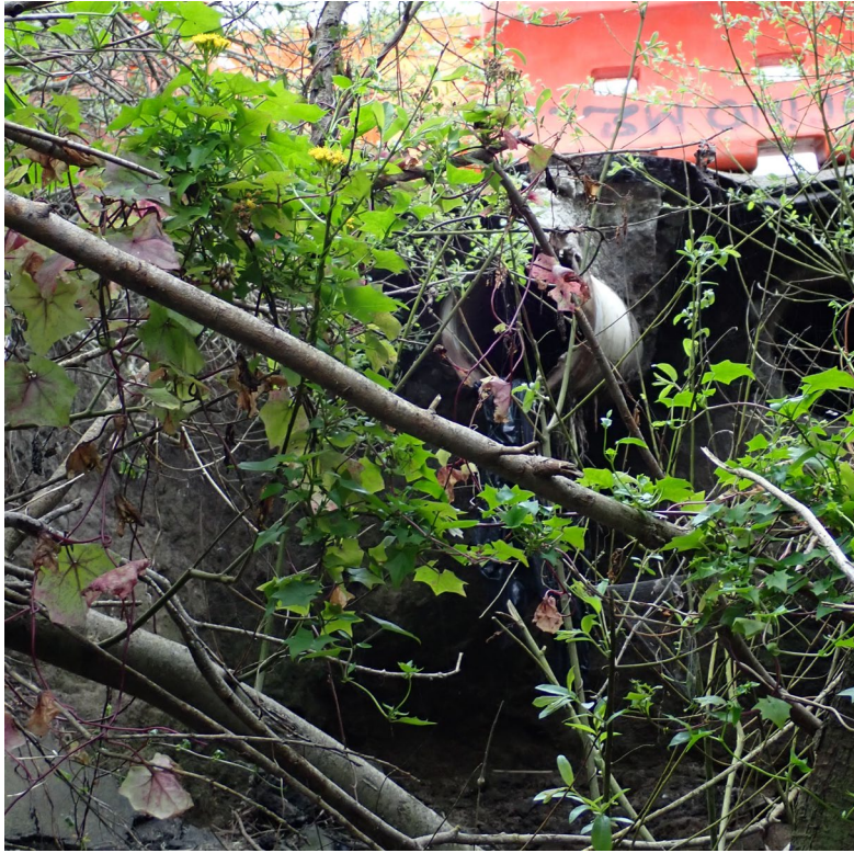
Figure 17 Outlet from parallel 17" and 24" culverts under Coastal Trail
