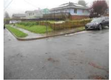
Photo 12 - Larger Park stormwater flow flooding into pseudo storm drain at end of Santa Maria at intersection with The Alameda
