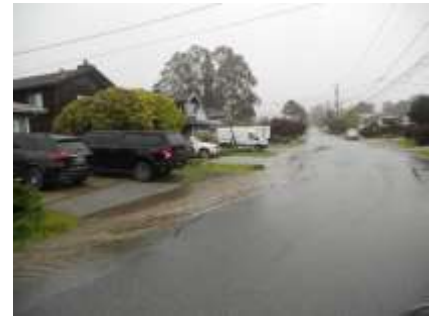
Photo 65 - Flooding on Sonora from stormwater pooling at the curve back to the storm drain
