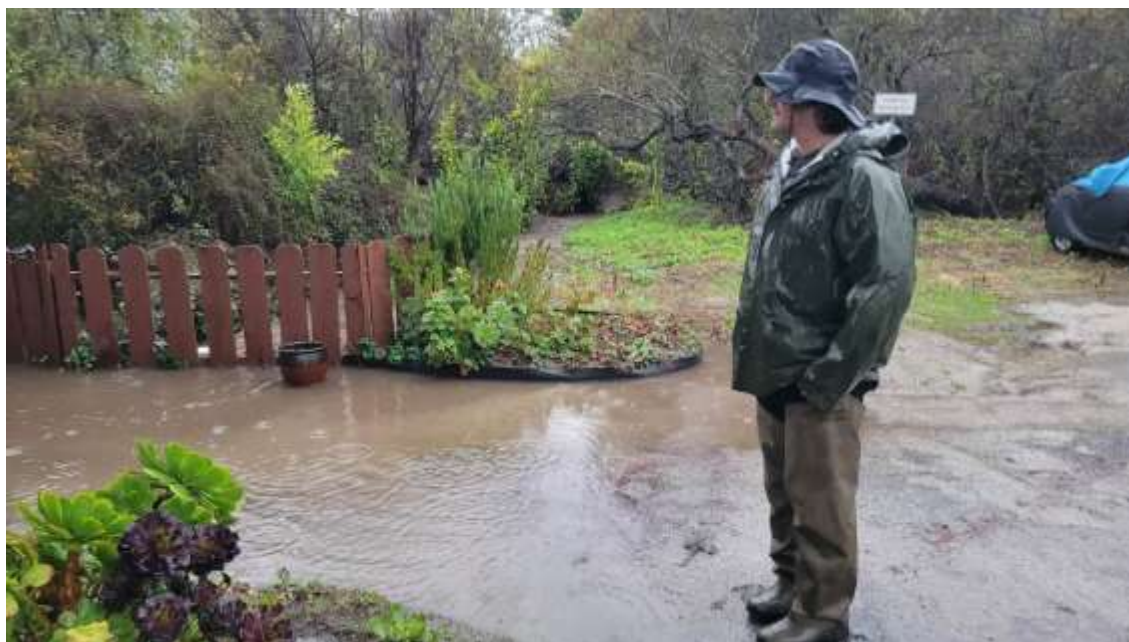
Photo 2. Creek overflow flooding driveway, yard and garage at 280 Kanoff Street. View is looking west (downstream). Photo date: 11-22-2024.
