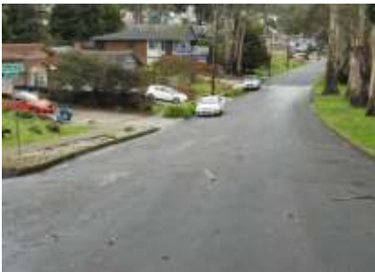
Photo 51 - Flooding down The Alameda from the convergence of Ave. Del Oro & San Carlos runoff
