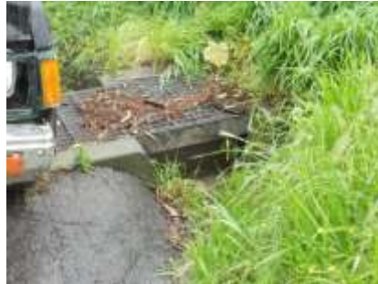
Photo 36 - Culvert in The Alameda's median
