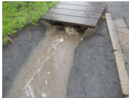
Photo 14 - Larger Park stormwater flow flooding from ditch into catch basin as entry into an underground storm system at The Alameda & Ave. Cabrillo
