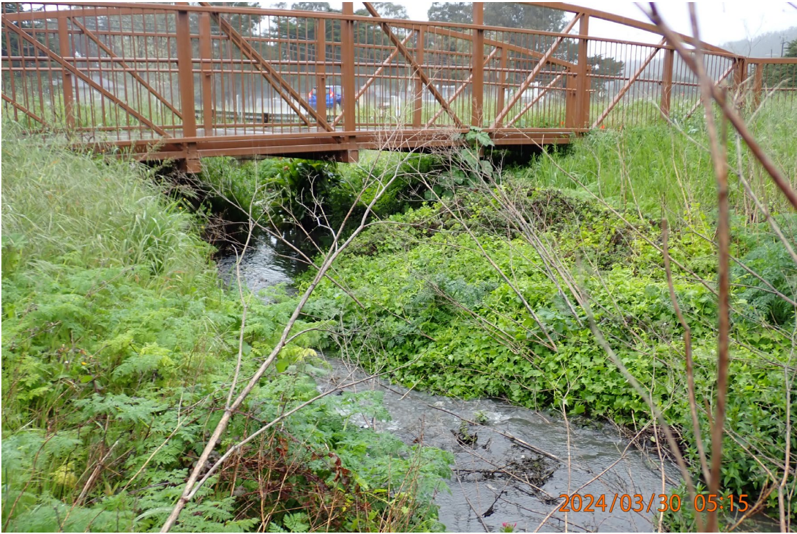
Figure 19 Pedestrian bridge northeast of Highway 1
