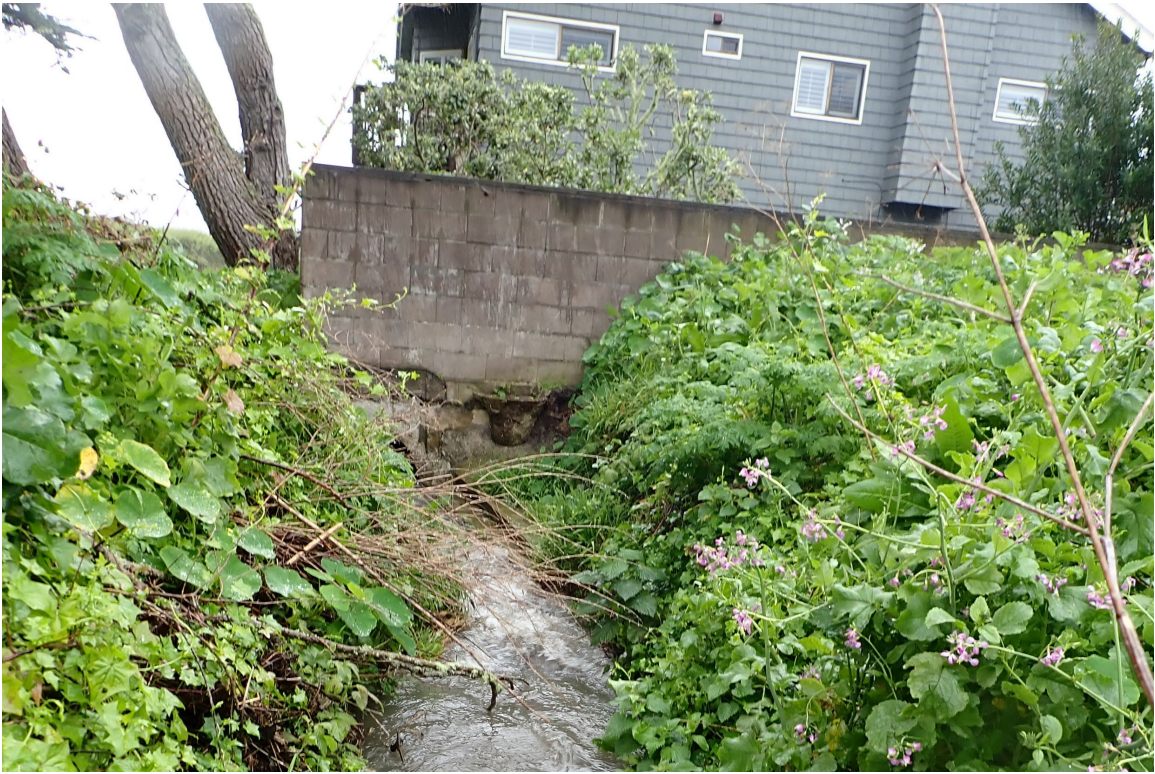
Figure 11 Inlet to 29" culvert under 2805 Naples Ave
