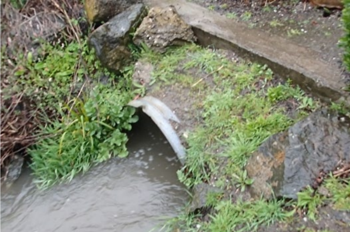
Figure 10 Outlet of 36" culvert under 2805 Alameda Ave
