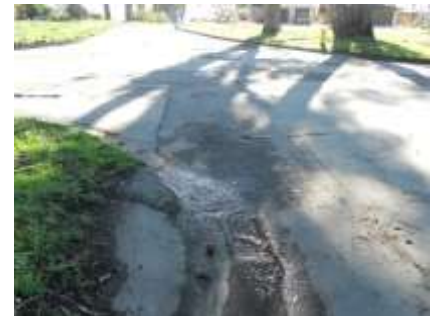
Photo 15 - Underground storm system from catch basin entry to manhole cover in Ave. Cabrillo at intersection with The Alameda
