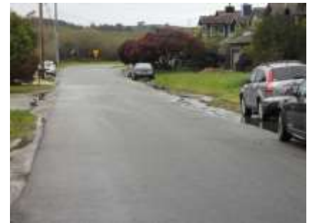
Photo 62 - Flooding down Sonora over x-street Presidio (towards storm drain)
