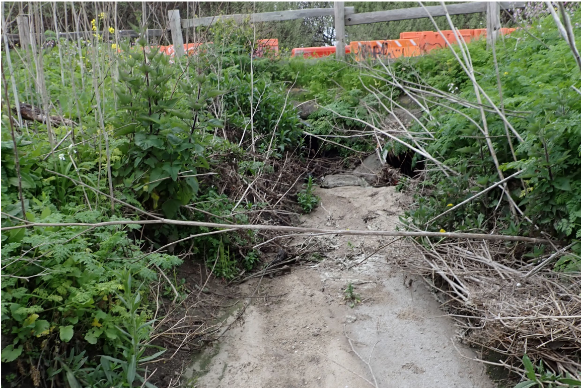
Figure 15 Inlet to parallel 17" and 24" culverts under Coastal Trail
