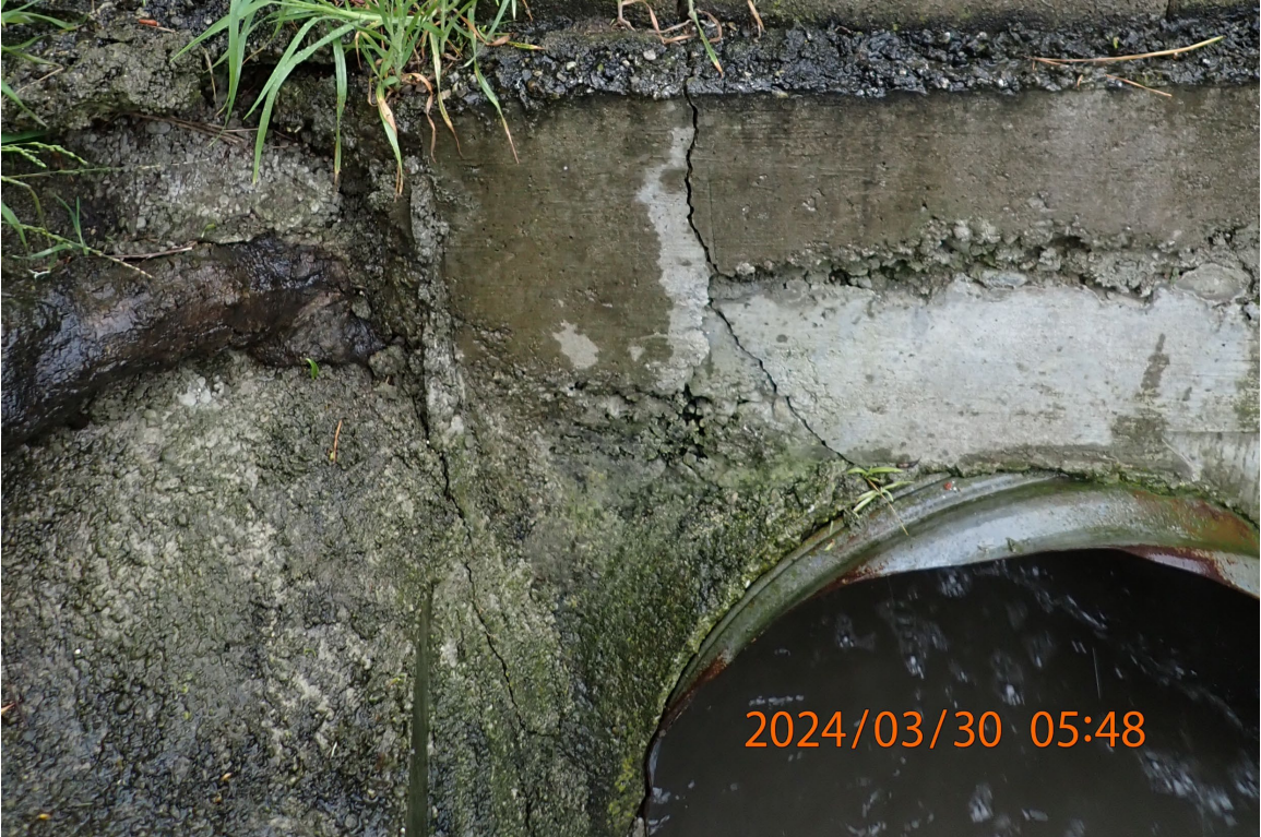
Figure 12 Inlet to 29" culvert under 2805 Naples Ave
