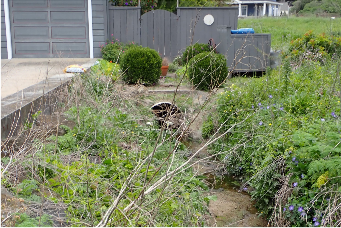
Figure 9 Outlet of 36" culvert under 2805 Alameda Ave
