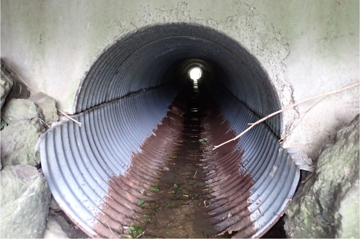
Figure 8 Inlet to 36" culvert under 2805 Alameda Ave
