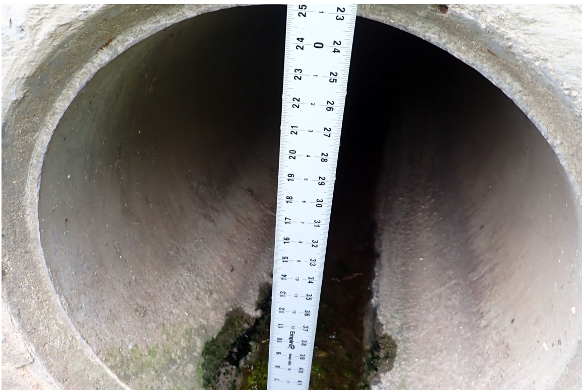
Figure 4 Inlet to one of the parallel 25" culverts under Highway 1
