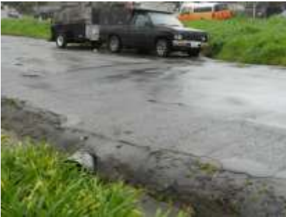
Photo 35 - Pipe under eastern side of The Alameda to culvert in median
