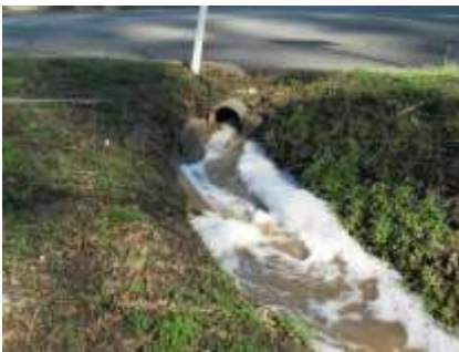
Photo 24 - Two stormwater drainage & runoff flows from pseudo storm drain under the eastern side of The Alameda to open-air ditch in its median
