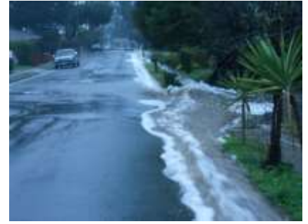
Photo 20 - Two stormwater drainage & runoff flows down Santa Maria over x-street Francisco
