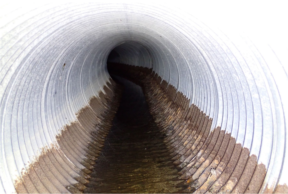
Figure 14 Interior of 29" culvert under 2805 Naples Ave, viewed from outlet
