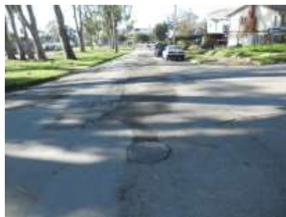
Photo 17 - Underground storm system down Ave. Cabrillo to its storm drain at Ave. Alhambra - from manhole cover at intersection with The Alameda
