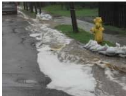
Photo 22 - Two stormwater drainage & runoff flows down Santa Maria at Palma
