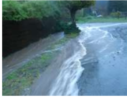
Photo 19 - Two stormwater drainage & runoff flows down Santa Maria
