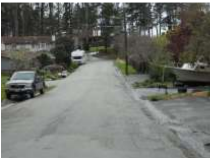
Photo 43 - Runoff down open-air ditches & under x-street Palma (looking down Ave. Del Oro)
