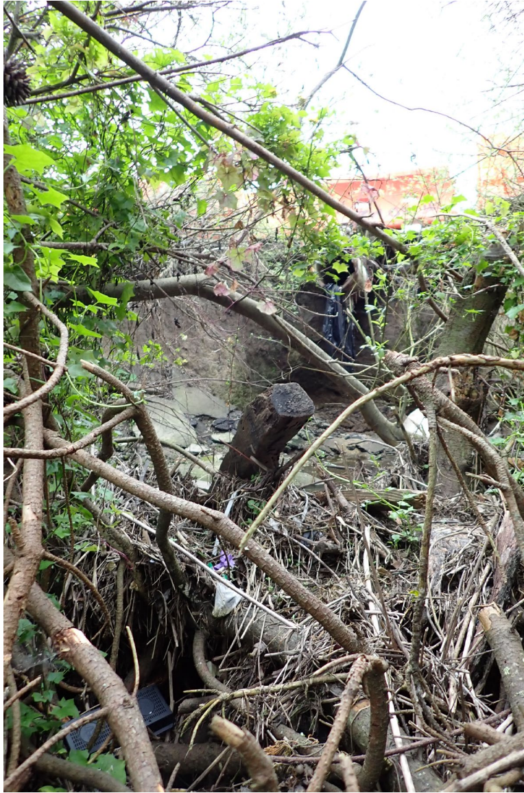
Figure 31 Outlet of Coastal Trail culverts, zoomed out to show drop
