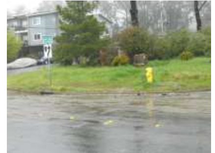
Photo 39 - Flooding down Ave. Portola to underground storm system storm drain at Ave. Alhambra
