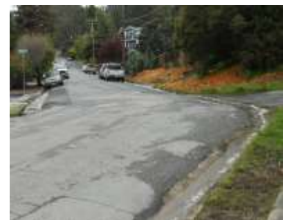
Photo 31 - Flooding down open-air ditches and over x-street Palma (looking up Ave. Portola)
