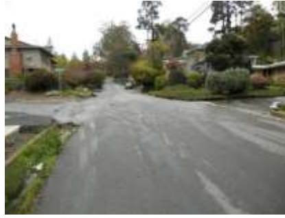
Photo 30 - Flooding down open-air ditches and over x-street Francisco (looking up Ave. Portola)
