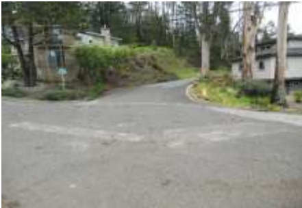
Photo 26 - Intersection of Ave. Portola & Columbus at Highlands
