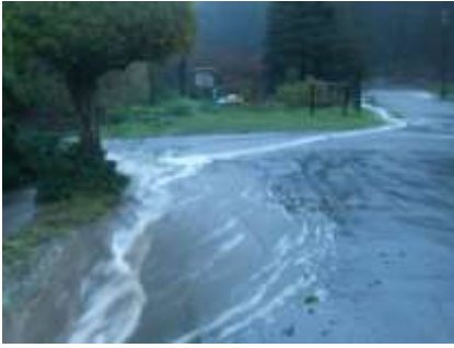
Photo 18 - Two stormwater drainage & runoff flows over intersection of Santa Maria & Columbus at Park entrance
