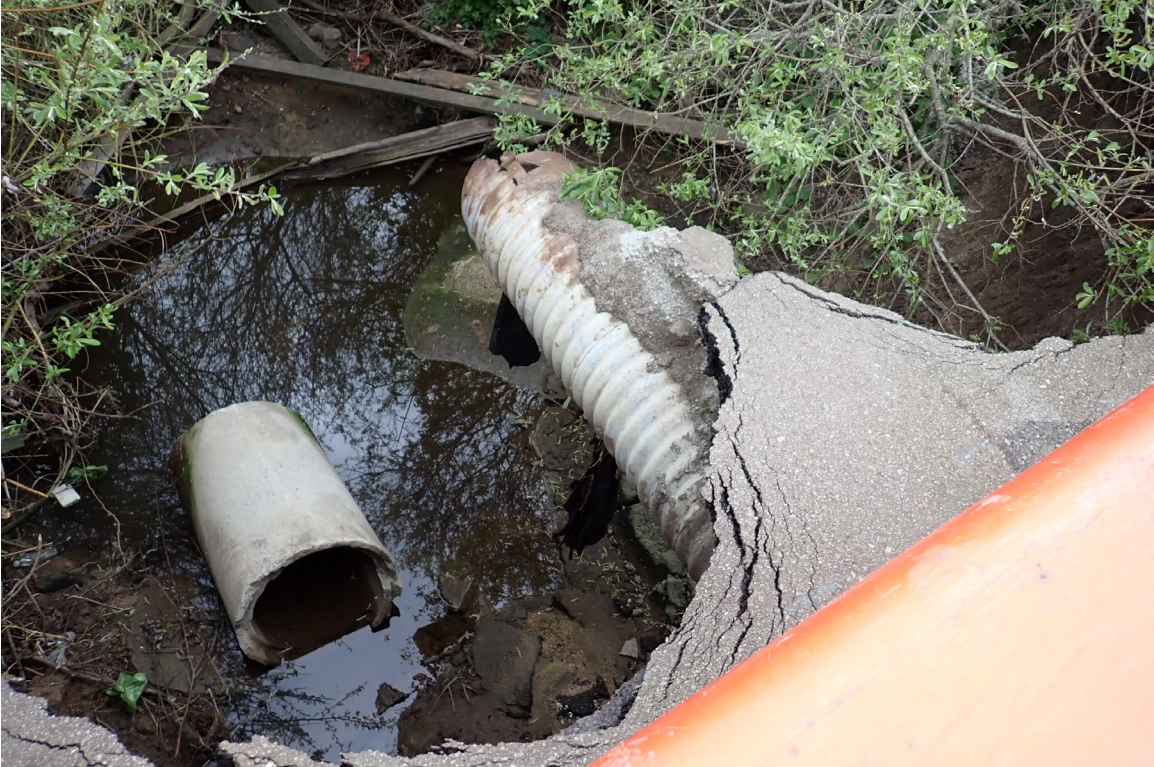
Figure 18 Outlet from parallel 17" and 24" culverts under Coastal Trail
