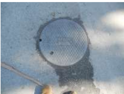
Photo 16 - Underground storm system manhole cover in Ave. Cabrillo at intersection with The Alameda
