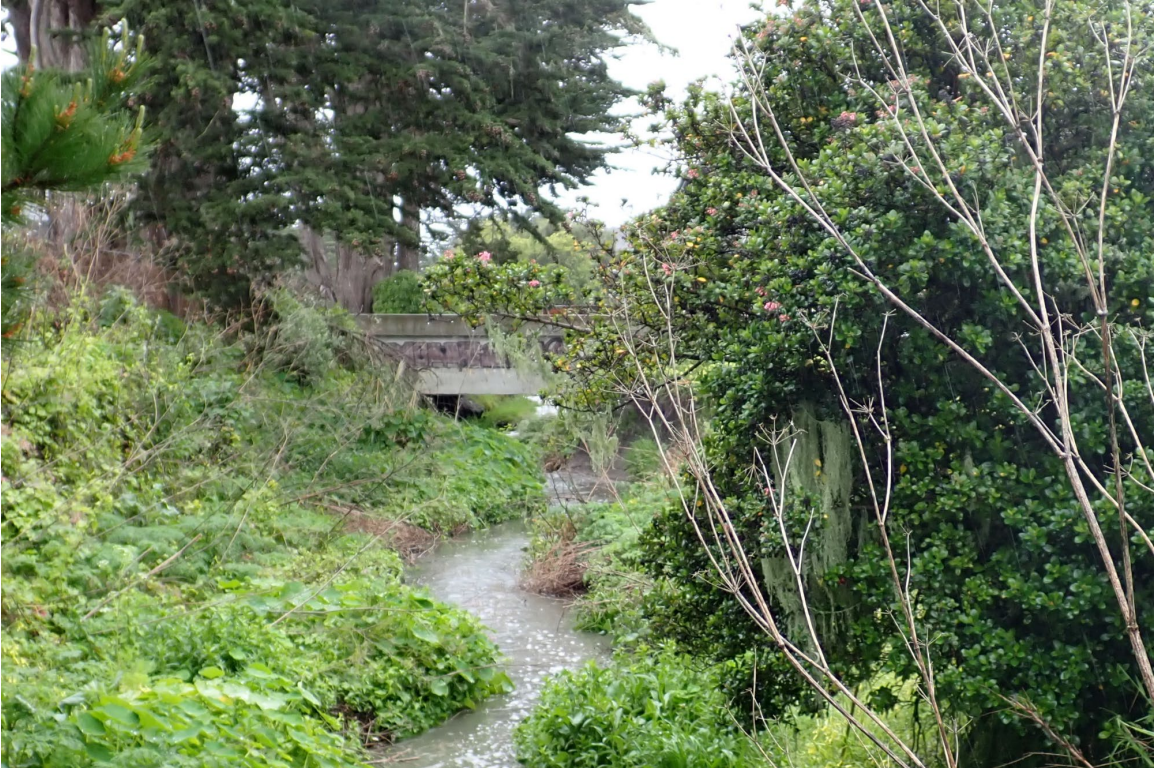
Figure 20 Pedestrian bridge at Pullman Ave
