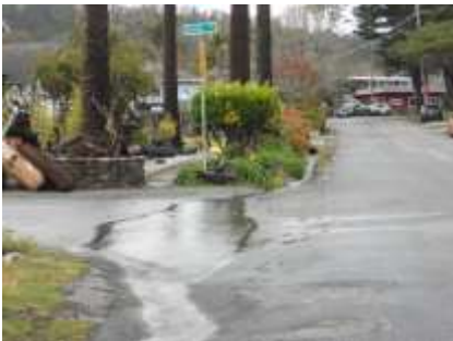
Photo 60 - Flooding down Sonora over x-street Sevilla (towards Ave. Granada)
