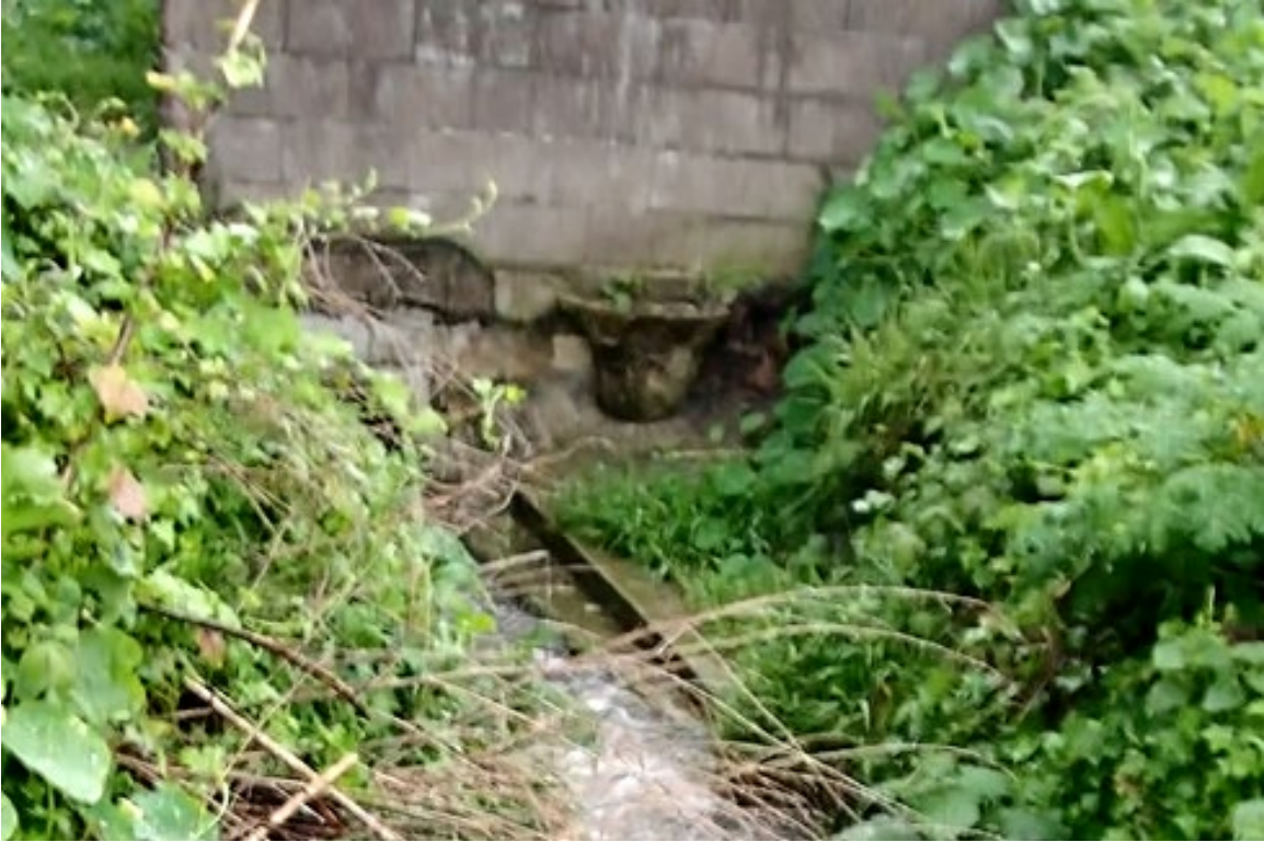
Figure 26 Concrete bank wall upstream of 2805 Naples Ave
