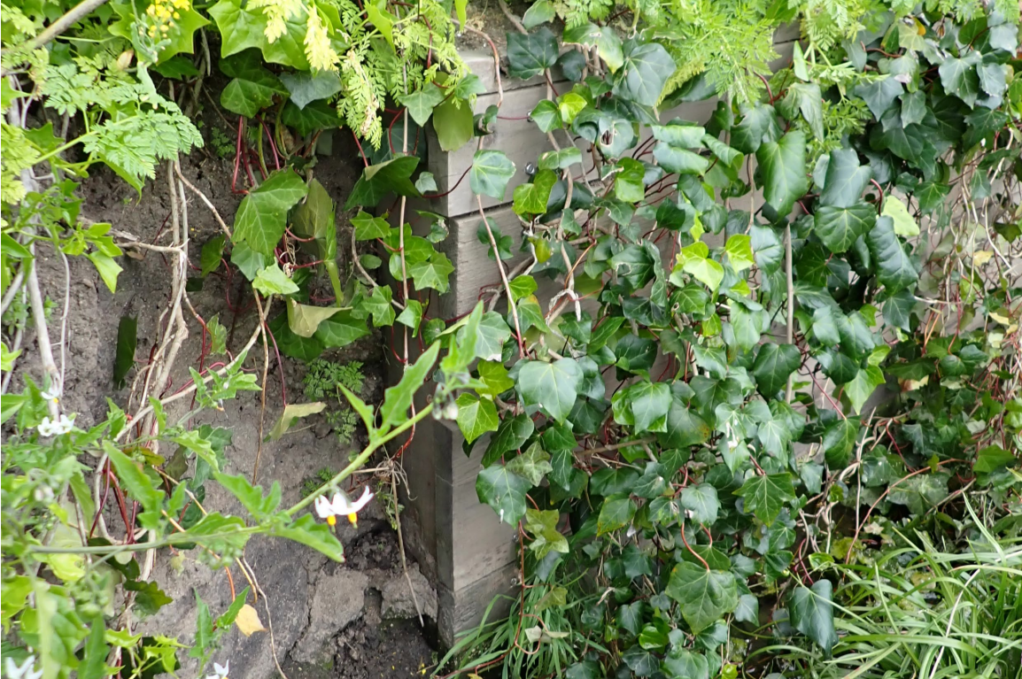
Figure 28 Timber retaining wall downstream of 2805 Naples Ave, downstream end
