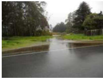
Photo 67 - Large pooling of stormwater runoff behind homes flooding onto Sonora beyond its curved portion (Coral Reef is to the left)
