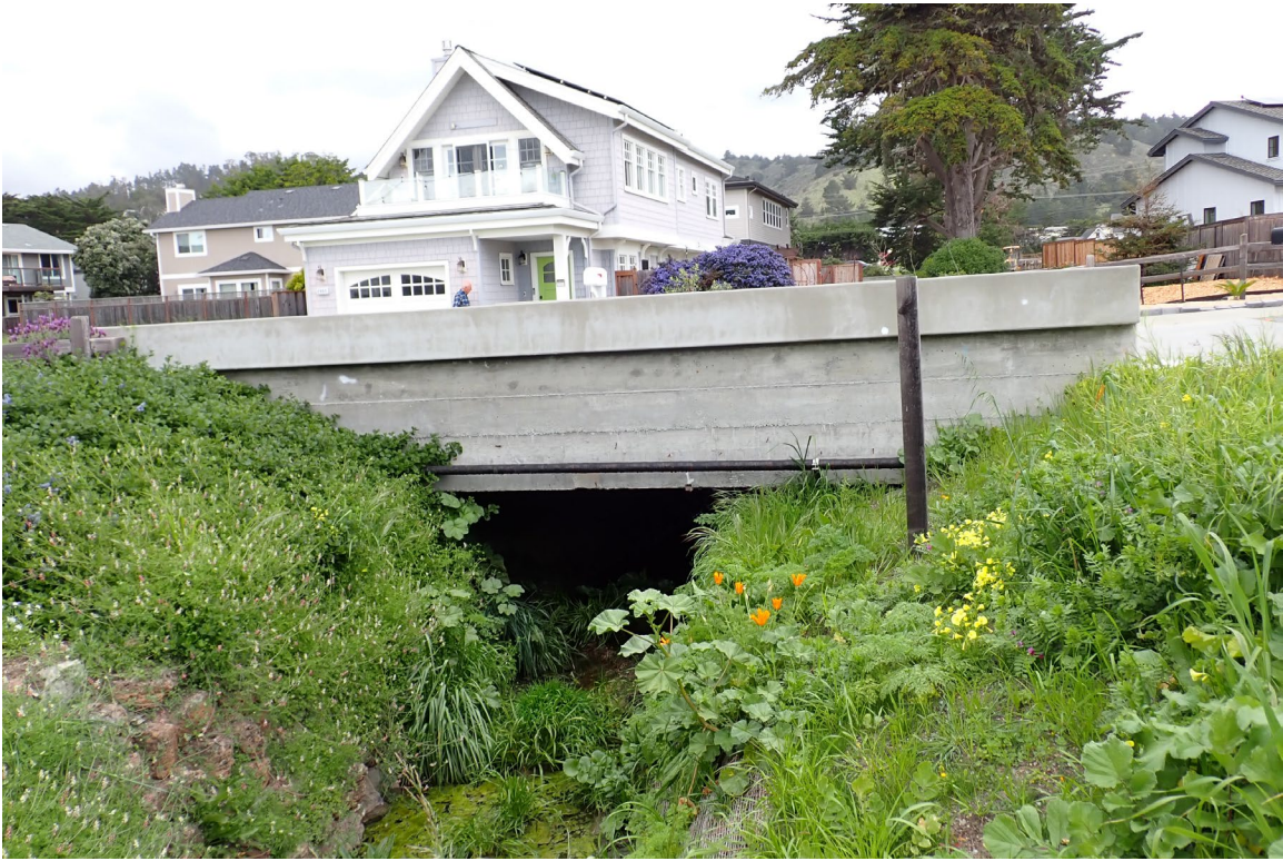
Figure 21 Pedestrian bridge at Champs Elysée Blvd
