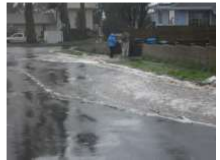
Photo 23 - Two stormwater drainage & runoff flows at Santa Maria end towards The Alameda into the pseudo storm drain
