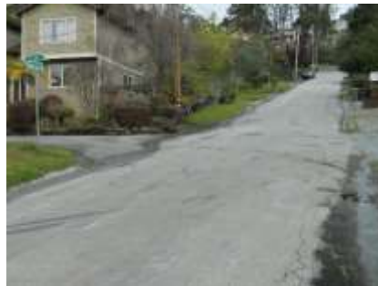
Photo 41 - Runoff down open-air ditches & over x-street Ferdinand (looking up Ave. Del Oro)
