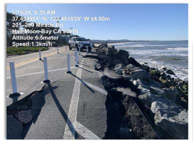
Photo examples of failed western edge of pavement (failed areas range in length and width).
