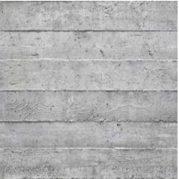
BOARD FORMED CONCRETE PLANTER
