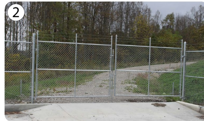
UTILITY FENCE AND VEHICULAR GATE
