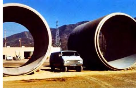
The nuclear reactors of SONGS units 2 and 3 are cooled by seawater that is taken in by large intake pipes and discharged back to the ocean via two diffuser lines
